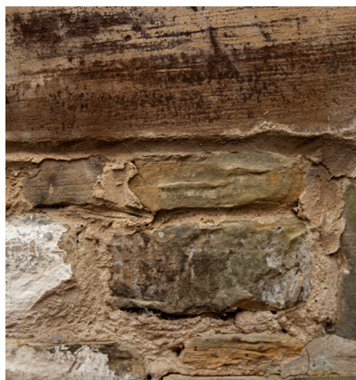
Fig 15 Recently quarried light riven faced ashlar showing slight rust coloured banding and fault line in horizontal bed. Photo copyright Stuart Page.
