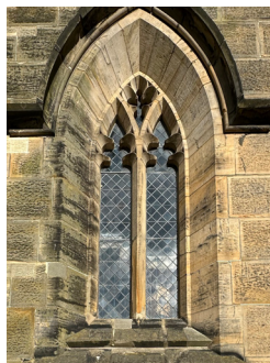
Figs 4 & 5 Holy Trinity Church, now Trinity Theatre and Arts Centre, with sandstone from the Calverley Estate quarries. This fine masonry is suffering from weathering at the mullion and cill junction (window detail right). Photos copyright Stuart Page.
