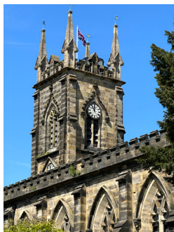
Figs 4 & 5 Holy Trinity Church, now Trinity Theatre and Arts Centre, with sandstone from the Calverley Estate quarries. This fine masonry is suffering from weathering at the mullion and cill junction (window detail right). Photos copyright Stuart Page.
