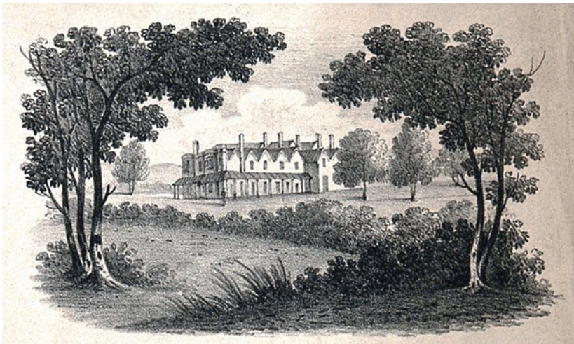
Figure 3. Mitchells, Burton's original design, north and east fronts.
