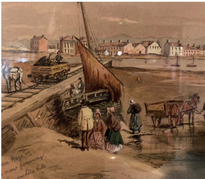
{5} - Building of the Railway Embankment 1839 by W.G. Herdman (Fleetwood Museum)
