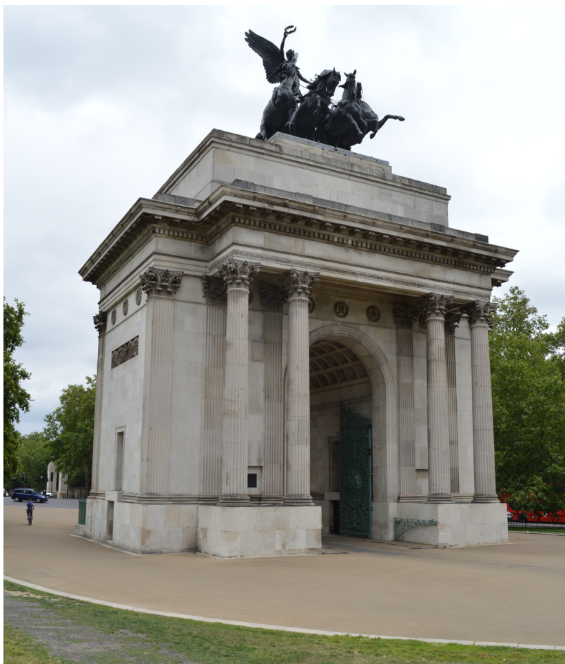
Fig 1. The Wellington Arch from the northwest, with reinstated fire exit on the left. Copyright Paul Avis
